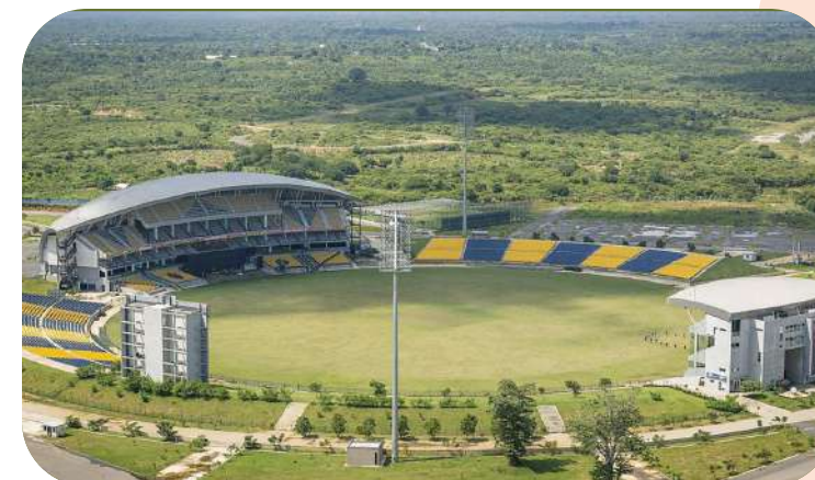
Sooriyawewa Cricket Stadium PA and BGM system
