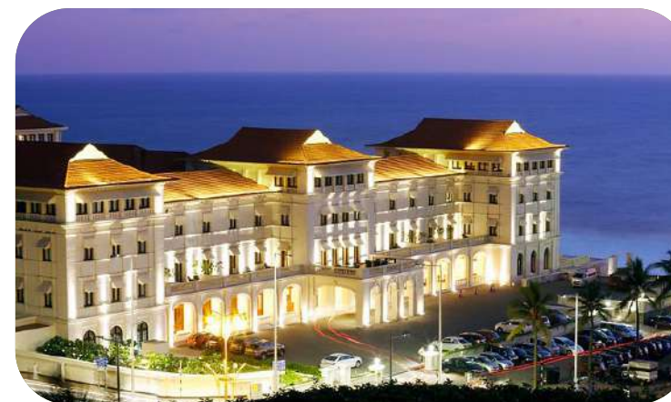
Galle Face Hotels Total Eaelectrical Services
