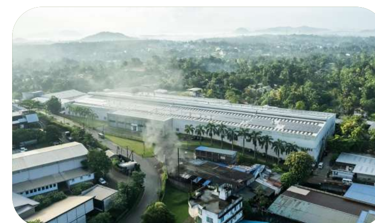
Lanka Tiles PLC CAPACITY: 550 KVA
