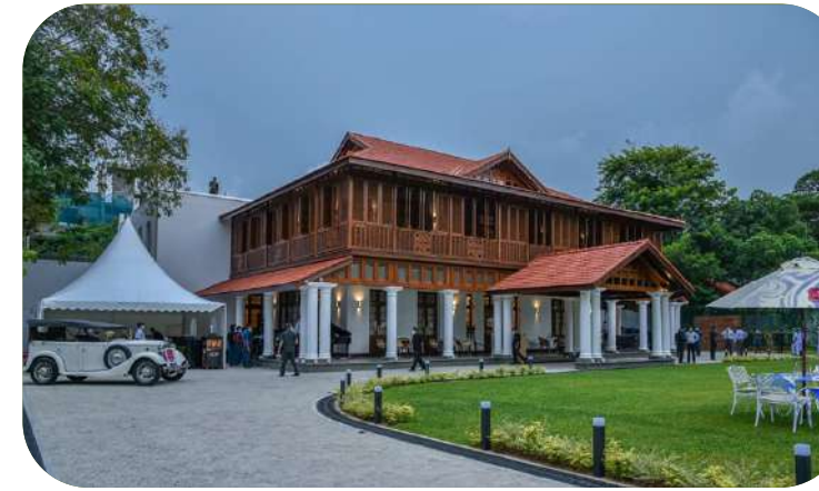
80 Club Total Plumbing Solution
