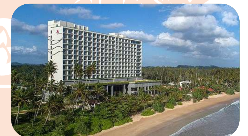
Marriot Resort & Spa Designing of Electrical Systems Winner of CIDA Award for installation excellence
