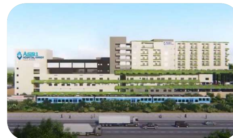
Asiri Hospitals Kandy Provision of Fire Protection Solutions
