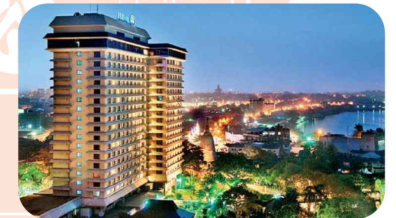
Hilton Colombo Total Plumbing Services
