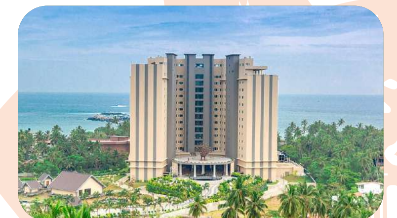
Araliya Unawatuna Luxury Resort Total Electrical Services
