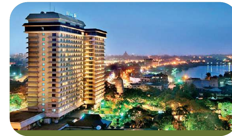
Hilton Colombo Central AC Chiller System
