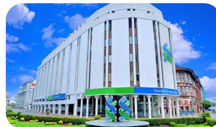
Standard Chartered Bank (for CBRE South Asias (Pvt.) Ltd.) Electrical Services | Mechanical Services Civil and Plumbing Services Building Management Services
