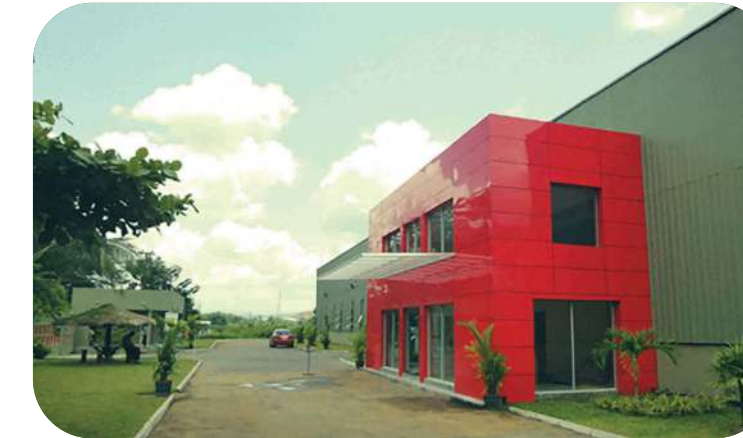
Orit Apparel, Lanka Supply of Pressure Pumps
