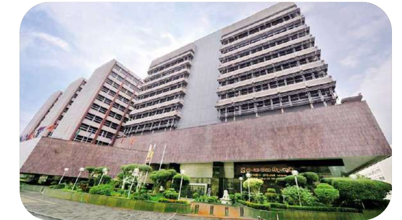
Central Bank of Sri Lanka Audio-Visual System for International Conference Hall at Head Office Building
