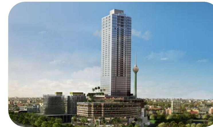
Colombo City Center PA System
