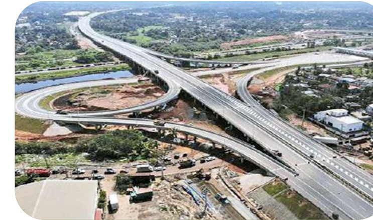
The Southern Expressway IPCCTV System with central monitoring station including the Network
