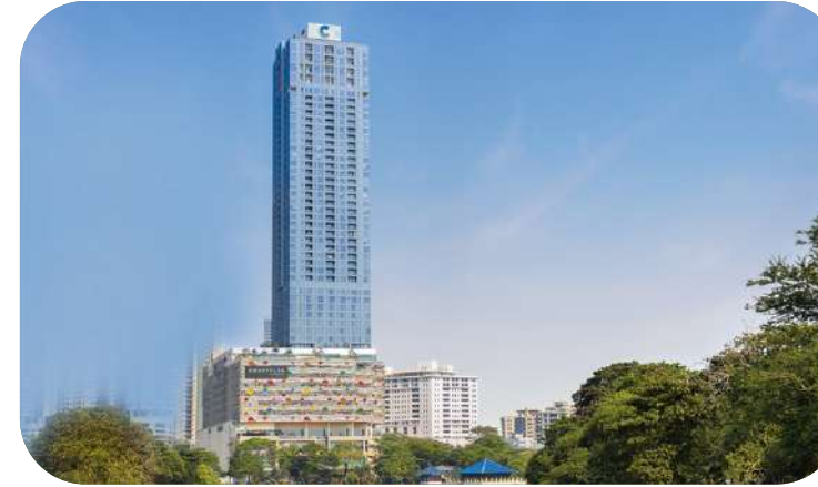
Colombo City Centre Total Electrical Services
