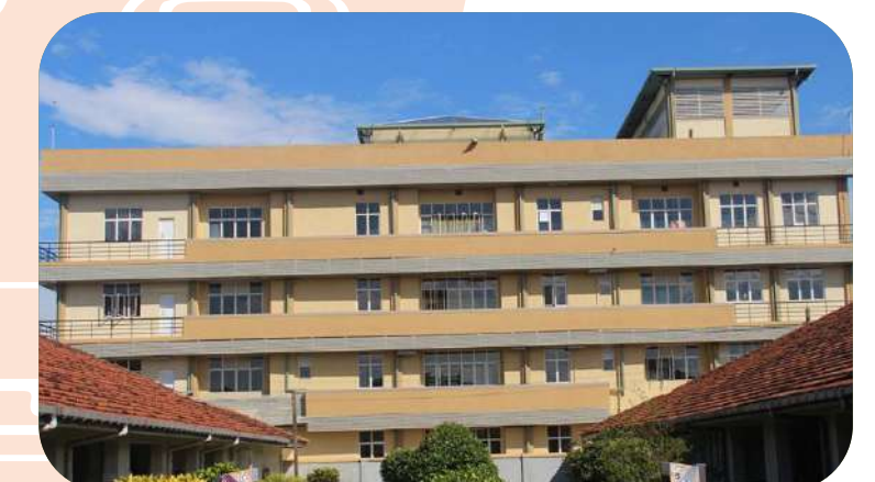
Castle Street Hospital Electrical services
