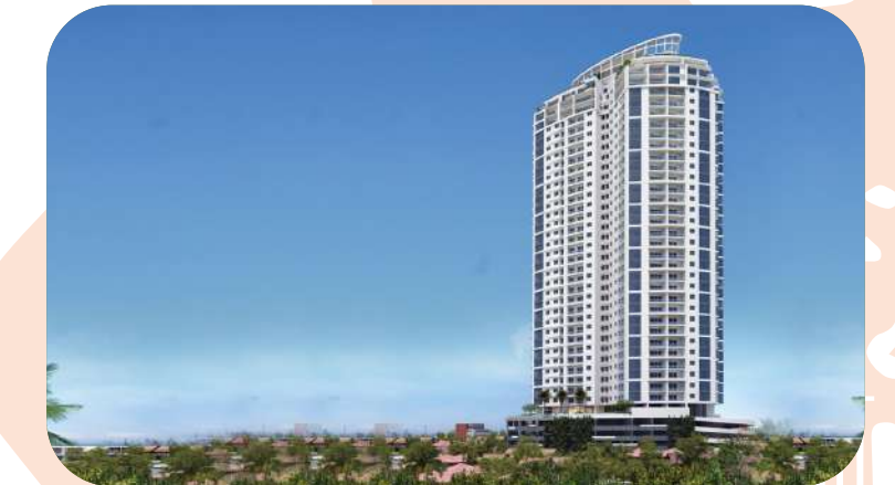
Capitol Heights Luxury Apartments Provision of Fire Protection Solutions
