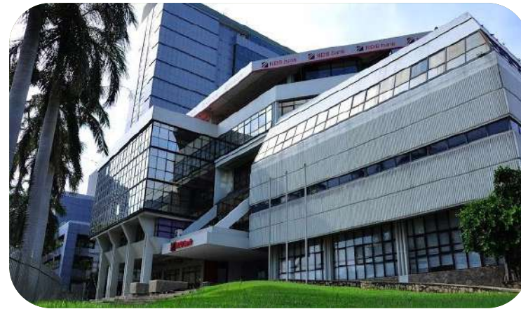
National Development Bank VRV System
