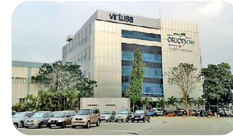
Virtusa Corporation CAPACITY: 840 KVA
