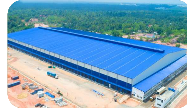
Camso Loadstar Warehousing and Logistics Facility Total Electrical Services
