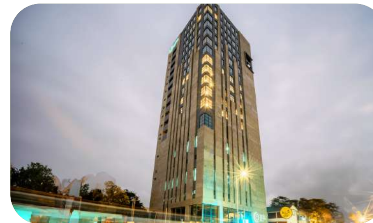
AOD Colombo Innovation Tower Total Plumbing Services
