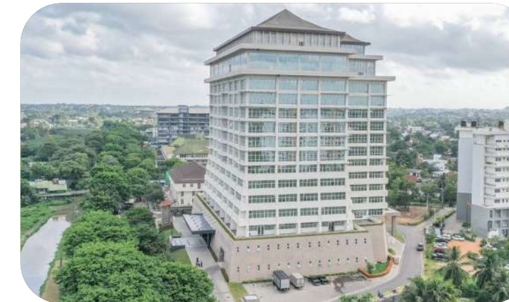
Western Provincial Council, Battaramulla LAN | Wi-Fi | PABX System for 3,000+ users
