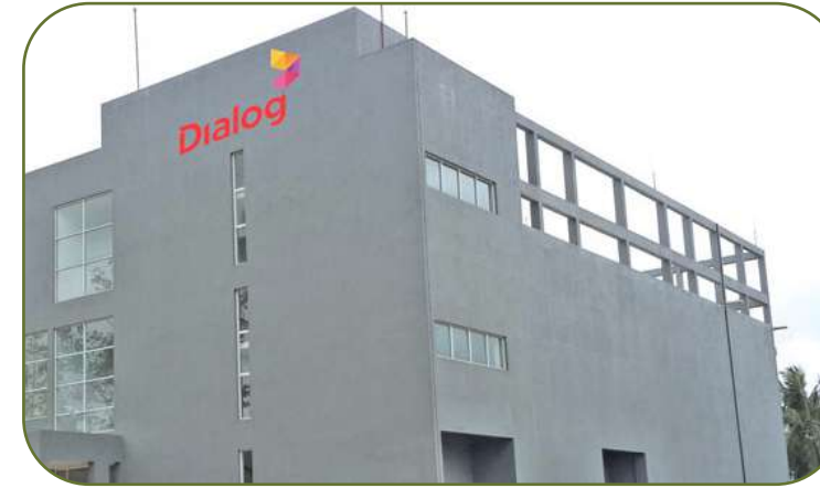
Dialog Data Centre Central AC Chiller System
