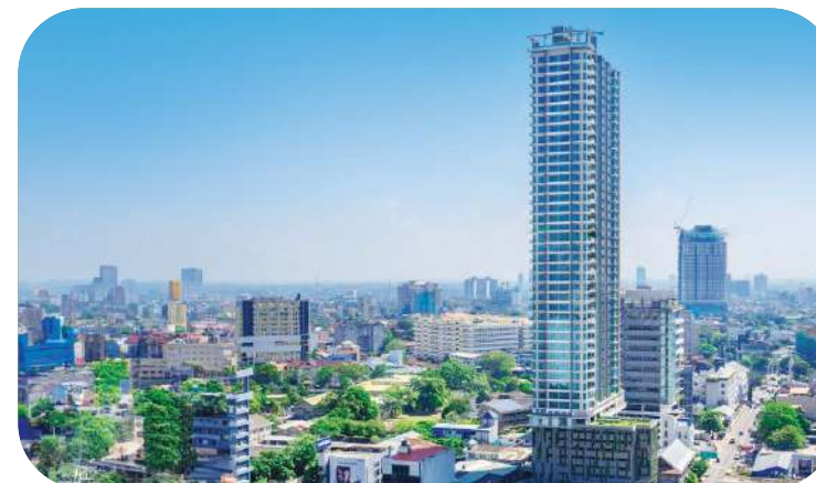
Union Place Apartments - Luna Towers PA and BGM system
