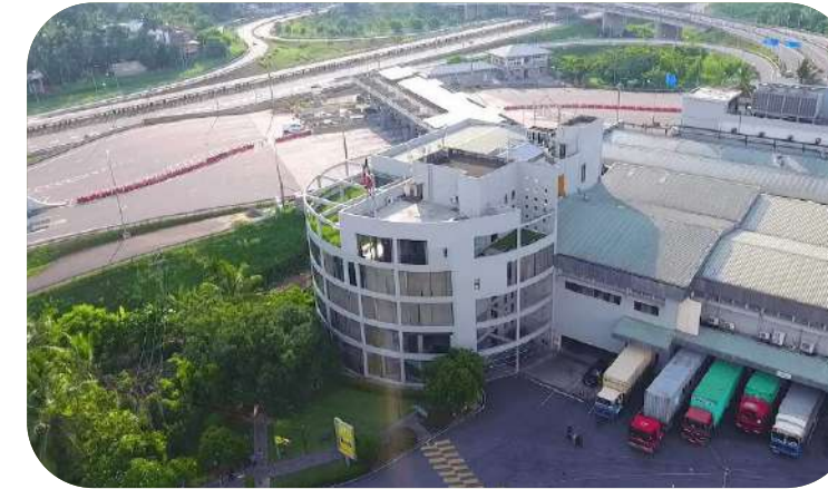
Ceylon Biscuit Limited CAPACITY: 1600 KVA
