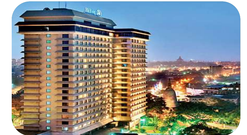
Hilton Colombo, Yala, Weerawila LAN, WIFI, PABX Firewall, Structured Cabling, 1500+ users
