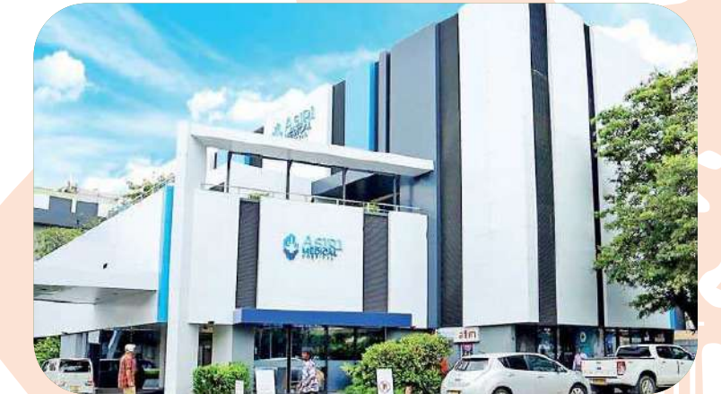
Asiri Hospital PLC CAPACITY: 280 KVA
