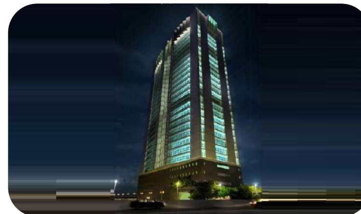
The Department of Labour - Head Office Integrated IPCCTV with over 160 cameras Access control system with over 110 doors Public address
