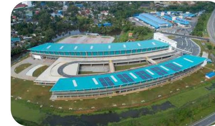
Manning Market Relocation Project Provision of Fire Protection Solutions
