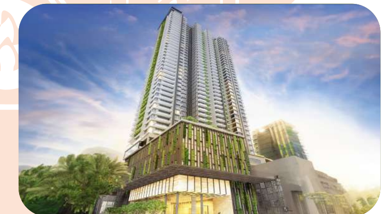
10.447 Luna Tower IPCCTV, PA, Video Door Phones, Vehicle barrier & lift access control
