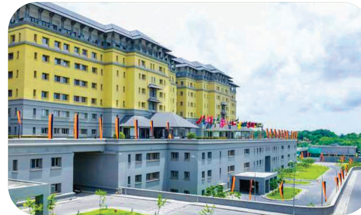
Ministry of Defense (Block 1/2) LAN, FIREWALL, PABX, UPS, NOC 1500+ users
