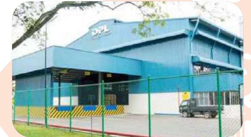
DPL Premier Gloves Pvt Ltd Provision Supply of Booster, Submersible and Fire Pumps
