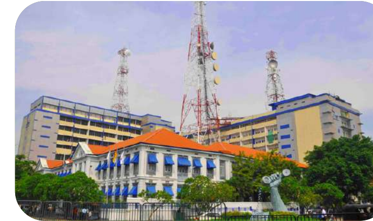
Sri Lanka Telecom Ruckus Wi-Fi | Data centre | UPS
