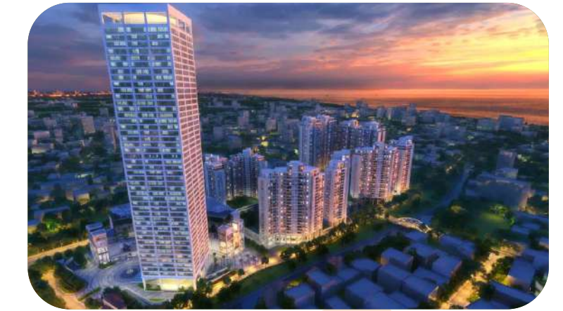
HSBC Mireka Tower Project Total Plumbing services
