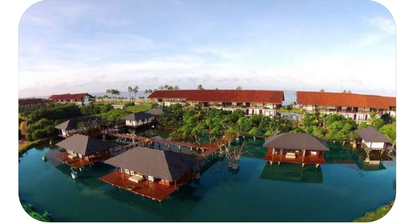
Ananthaya Resort and Spa, Chilaw Total Electrical Services
