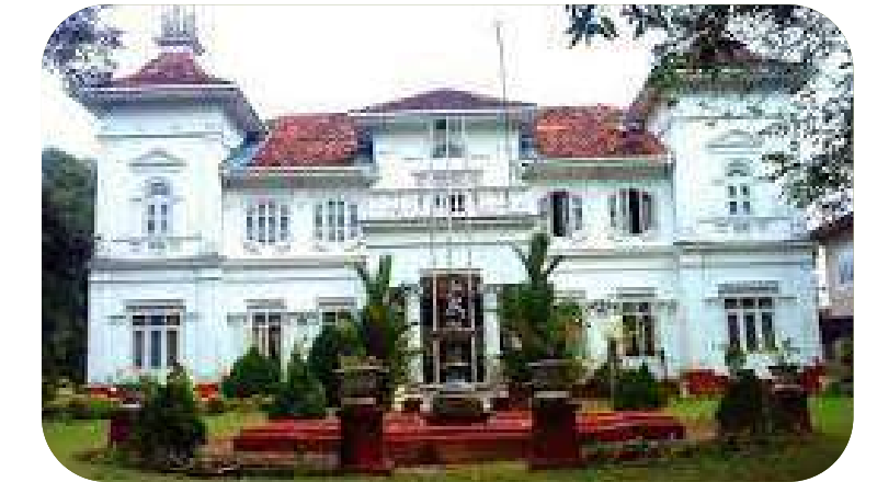
District Secretariat Office Gampaha LAN, WIFI, Firewall, PABX, Structured Cables 600+ Users
