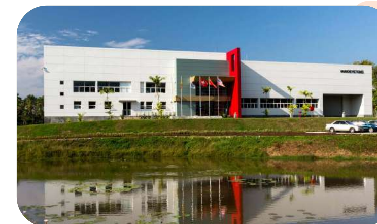
Vario Supply of Water Pumps
