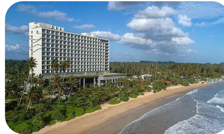
Weligama Bay Marriott Resort & Spa 198 Room hotel with total LAN Passive network with 885 nodes
