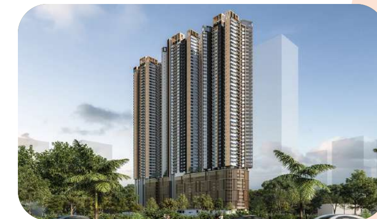
Trizen Apartment Tower 02- total plumbing system Installation
