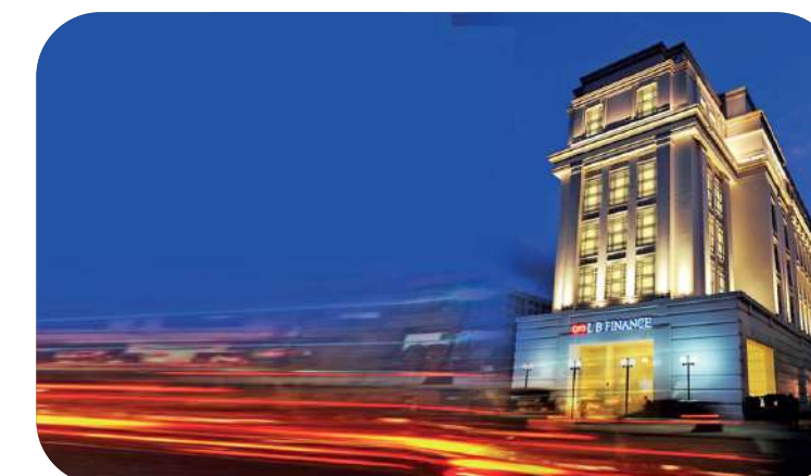
LB Finance Electrical Services | Mechanical Services Carpentry Services
