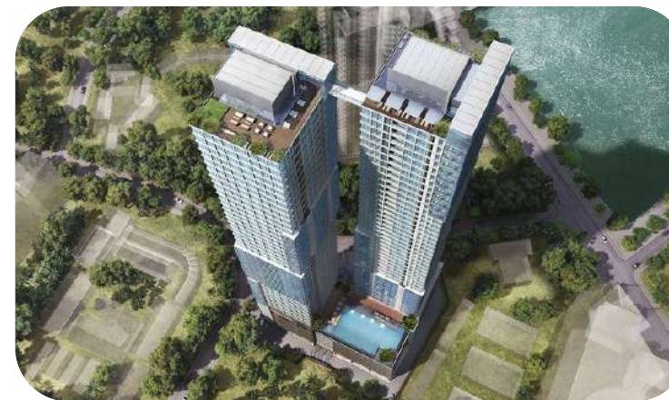
Capitol TwinPeaks Total Electrical Services
